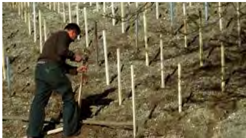
Planting: setting up of the vine stakes
